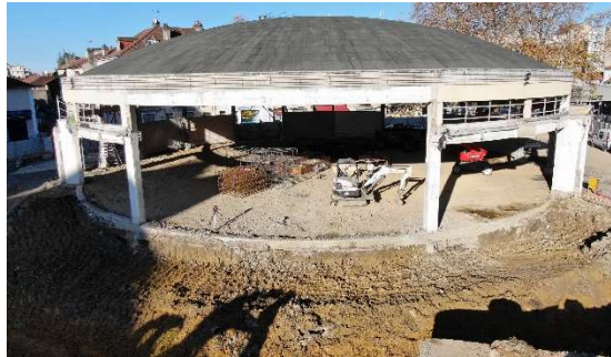
Le Foirail in Pau before installation of the gantry
