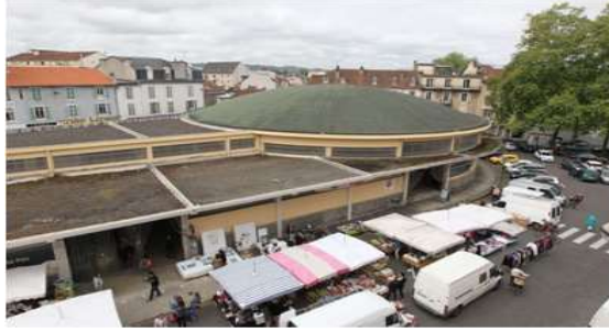
Le Foirail in Pau before demolition
